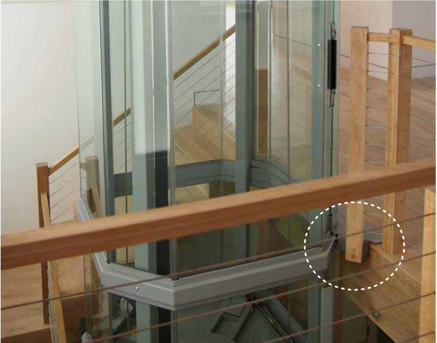
Figure 25: Balcony plate and handrail information - octagonal glass (OGM) type 1
